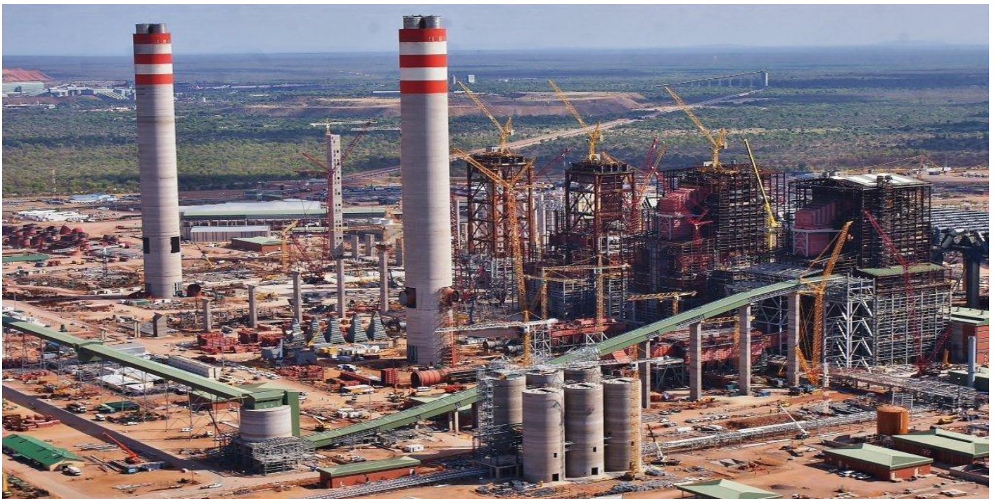
Figure 1: Construction at Medupi Power Station
